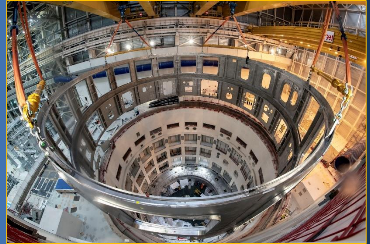
Inserting the Cryostat Lower Cylinder into the Tokamak Pit, 31 August 2020
